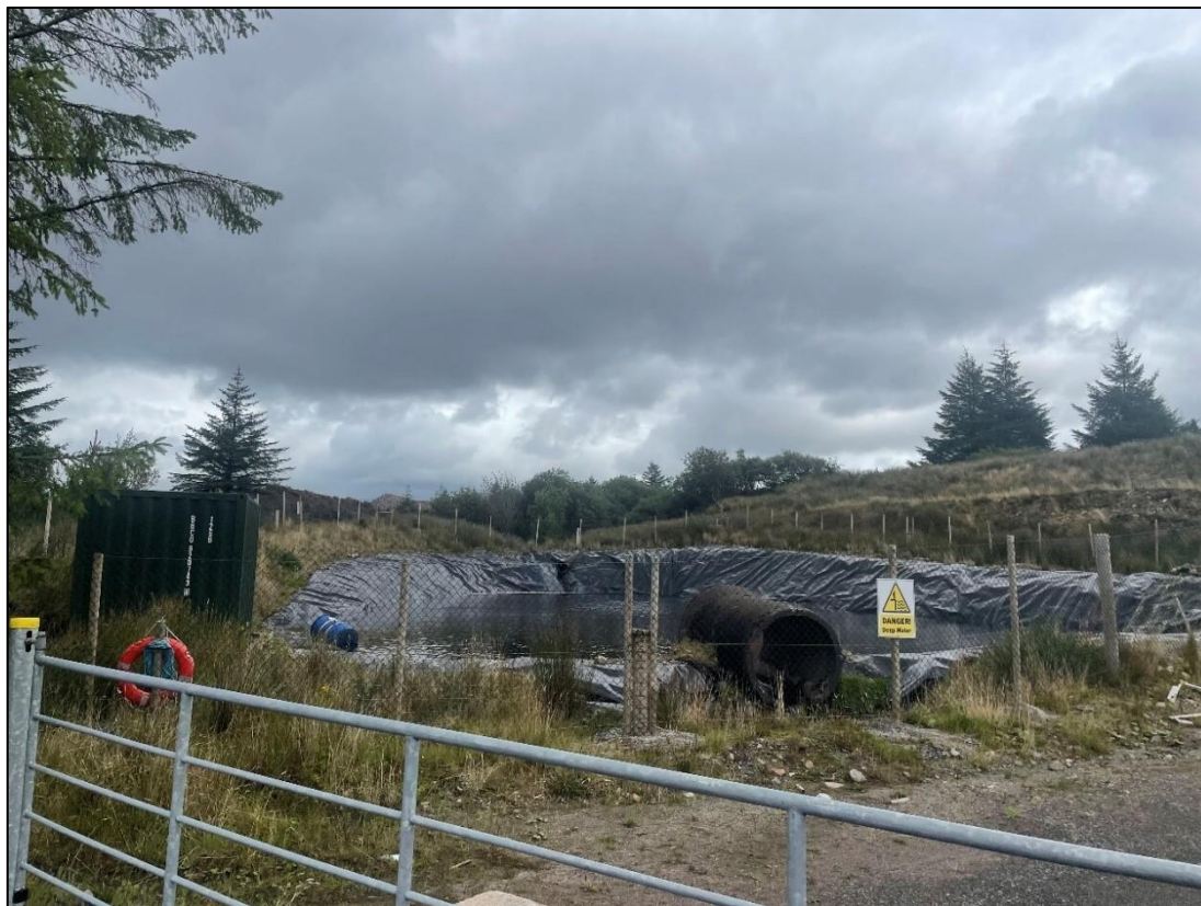
Plate 6-14 Artificial Pond close to the quarry entrance - lined as part of the Existing Development
