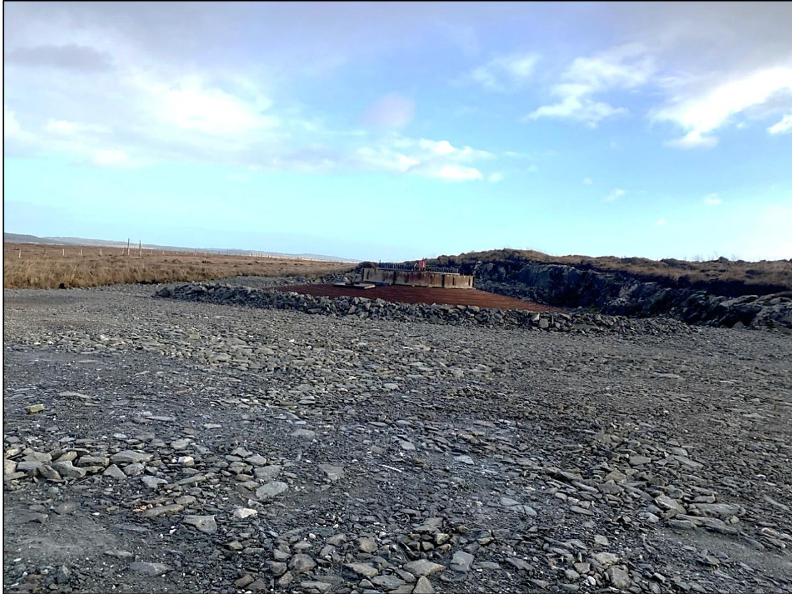
Plate 6-5 Representative photo of the wind farm infrastructure at T19, which is similar at T16
